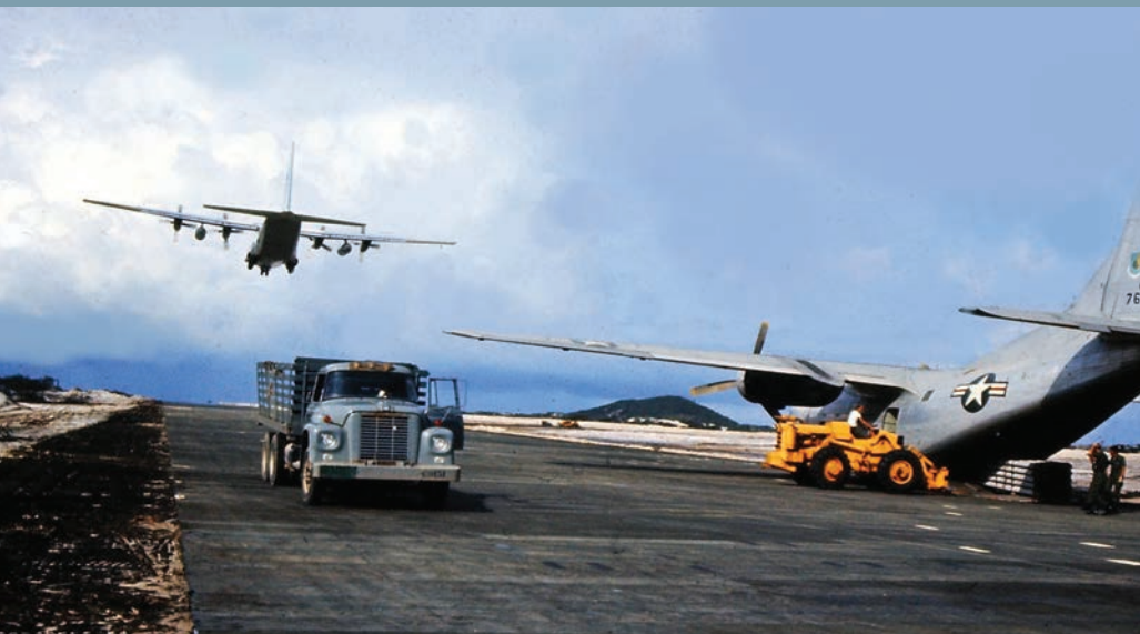
While building Cam Ranh Bay runway Provider unloads aluminium planking as C-130E lands long. (Photo courtesy of R.C. Weaver)
