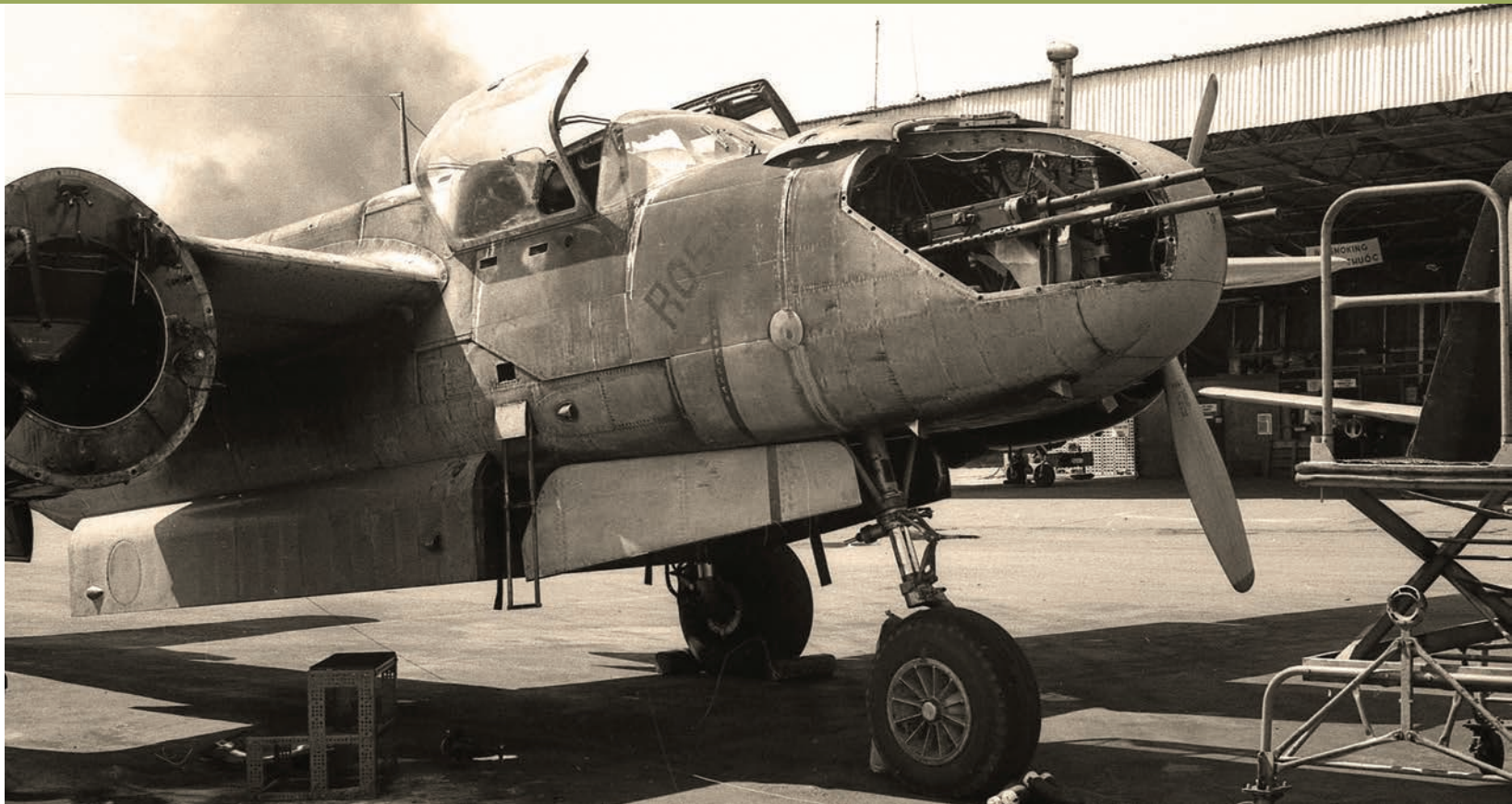
Rosie was a typical Farm Gate B-26. Little was known of her history. She was just a tired old veteran of several wars, in need of a wash job. Here she takes time off for an engine change and never-ending maintenance to her .50 caliber machine guns. (Photo by Maurice Bourne)
